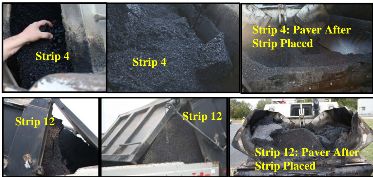
Figure 5.7. Conglomerates of Mix at Longer Haul Times
