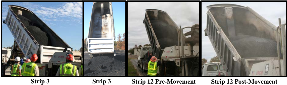
Figure 5.6. Removal of Mix From Trucks for Longer Haul Times
