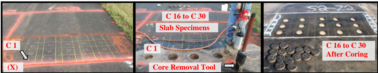
Figure 3.23. Marking and Removing Cores
