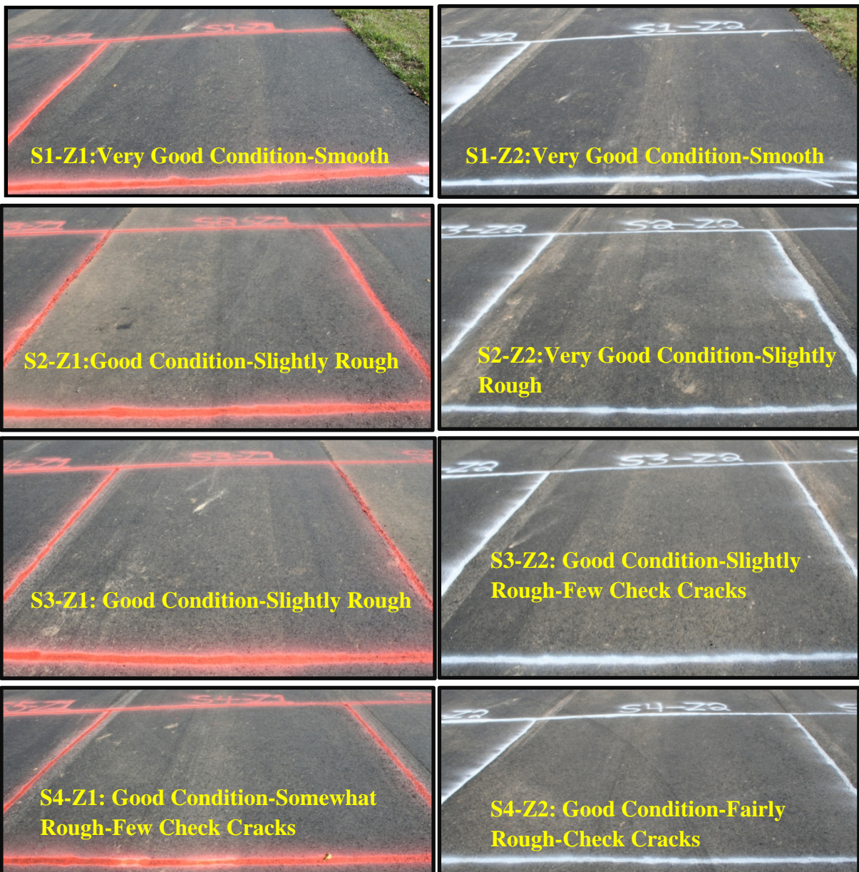
Figure 5.8. Visual Evaluation of Strips 1 to 4 (HMA) Post Construction
