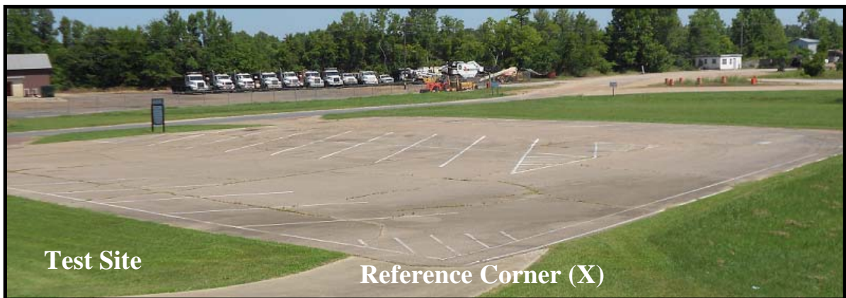
(a) Photograph of Test Site on June 30, 2011 prior to crack cleaning
