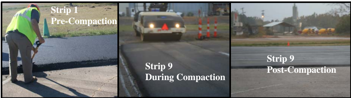
Figure 5.3. Representative Site Conditions During Paving
