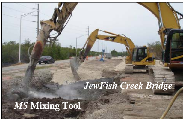
Figure 4.6. Mass Stabilization (MS) and Column Stabilization (CS) Mixing Tools
