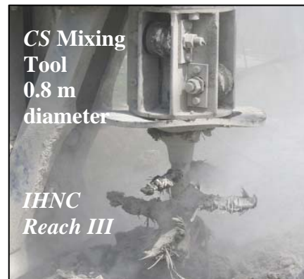
Figure 4.6. Mass Stabilization (MS) and Column Stabilization (CS) Mixing Tools
