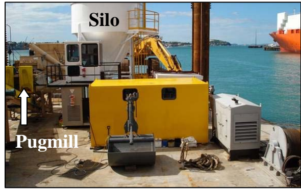
(b) Barge Mounted Pugmill
