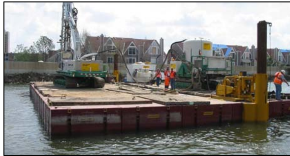
Figure 4.5. Barge Mounted Soil Mixing Equipment
