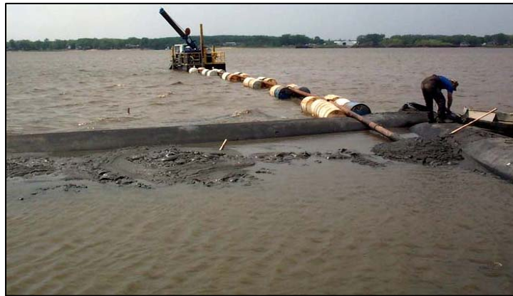
Figure 2.2. Beginning of Pumping Sediment for Pilot Scale Island Provided by ISTC
