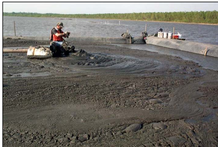
Figure 2.3. Nearing Completion of Pumping Sediment for Pilot Island Provided by ISTC
