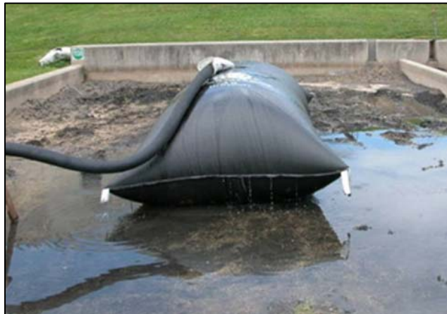
Figure 6.1. Pilot Scale Dewatering Test
