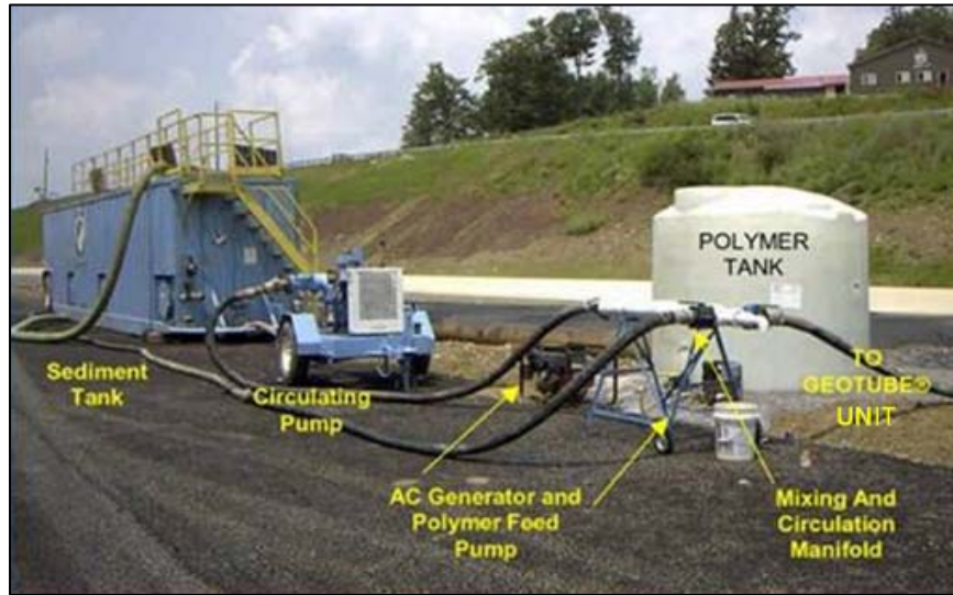
Figure 2.2. Example Polymer Dewatering System
