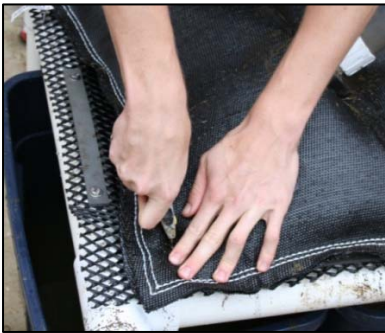
(c) Cutting of Pillow after Dewatering
