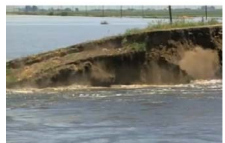
Photo by California Department of Water Resources
