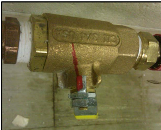
b) Water Shutoff Valve Setting
