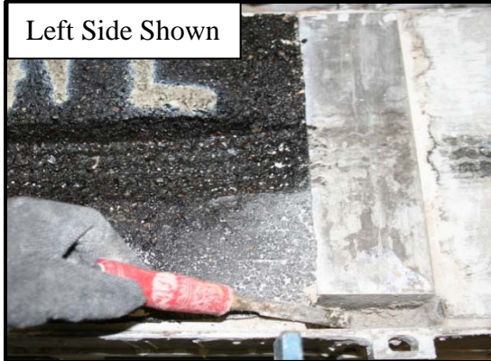
a) Grout Plug at End of Spacer Block
