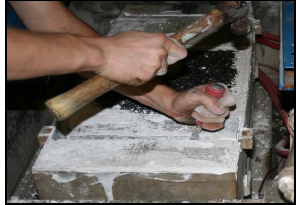
b) Grout in Front of Spacer Block
